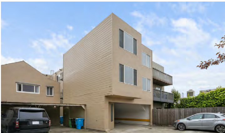
361-365 2nd Ave - Rear Yard
